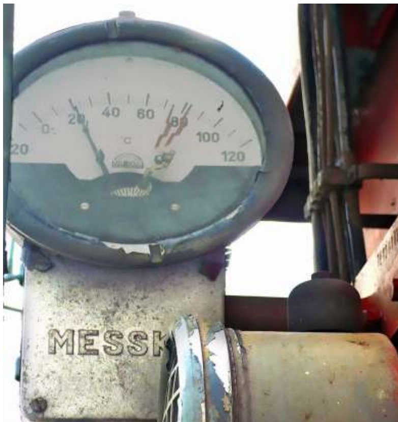
Figure 1 – Transformer thermometer
